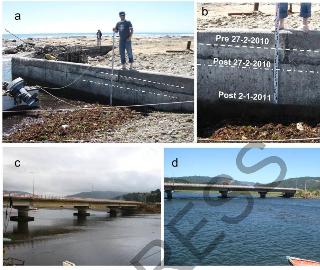
F9-11. Evidences of vertical changes at Mocha Island and Tirúa after Araucanía 2011 earthquake: a and b is the same place at Mocha Island shown in Fig. 7d. It is clear the sea level drop of 50 cm. c and d. Tirúa bridge. Left photo taken on April 27th 2010 one hour after the low tide. Right photo: same view on January 20th 2011 at the time of low tide. Note the upper position of the water in the columns evidenced 20 cm of subsidence after the Mw=7.1 event. The Tirúa River had more caudal on January 2011, even if we consider that this is the summer dry season.
